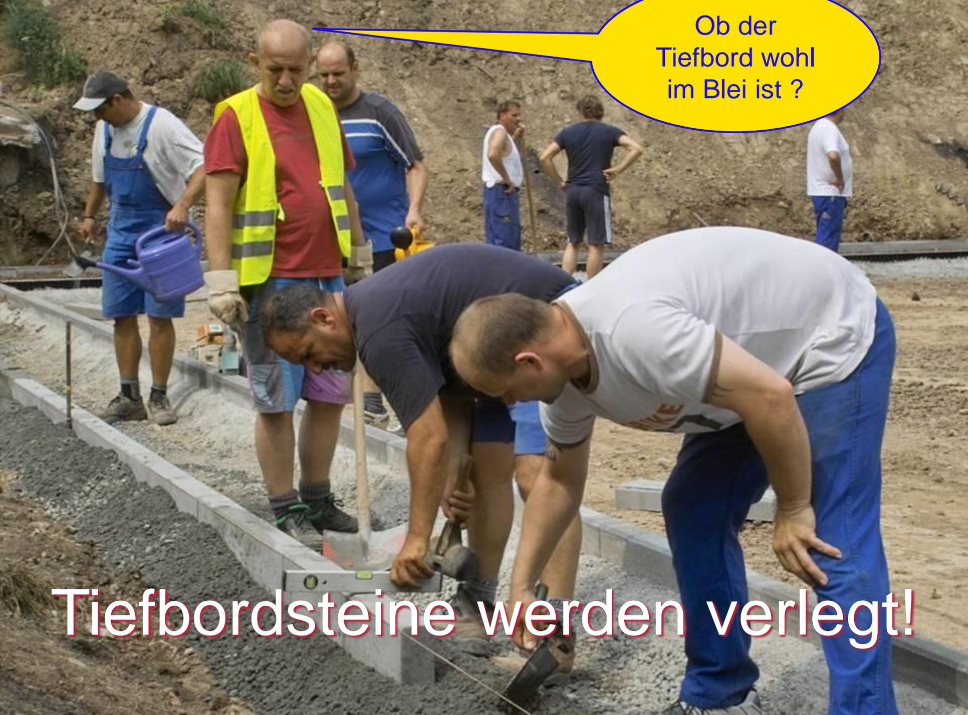
A group of construction workers are working on a hillside, laying concrete curb stones. In the foreground, two men are bent over, one using a mallet to tap a stone into place while the other holds a level. In the background, other workers are visible, some holding tools and others observing. The terrain is a mix of dirt and gravel.
