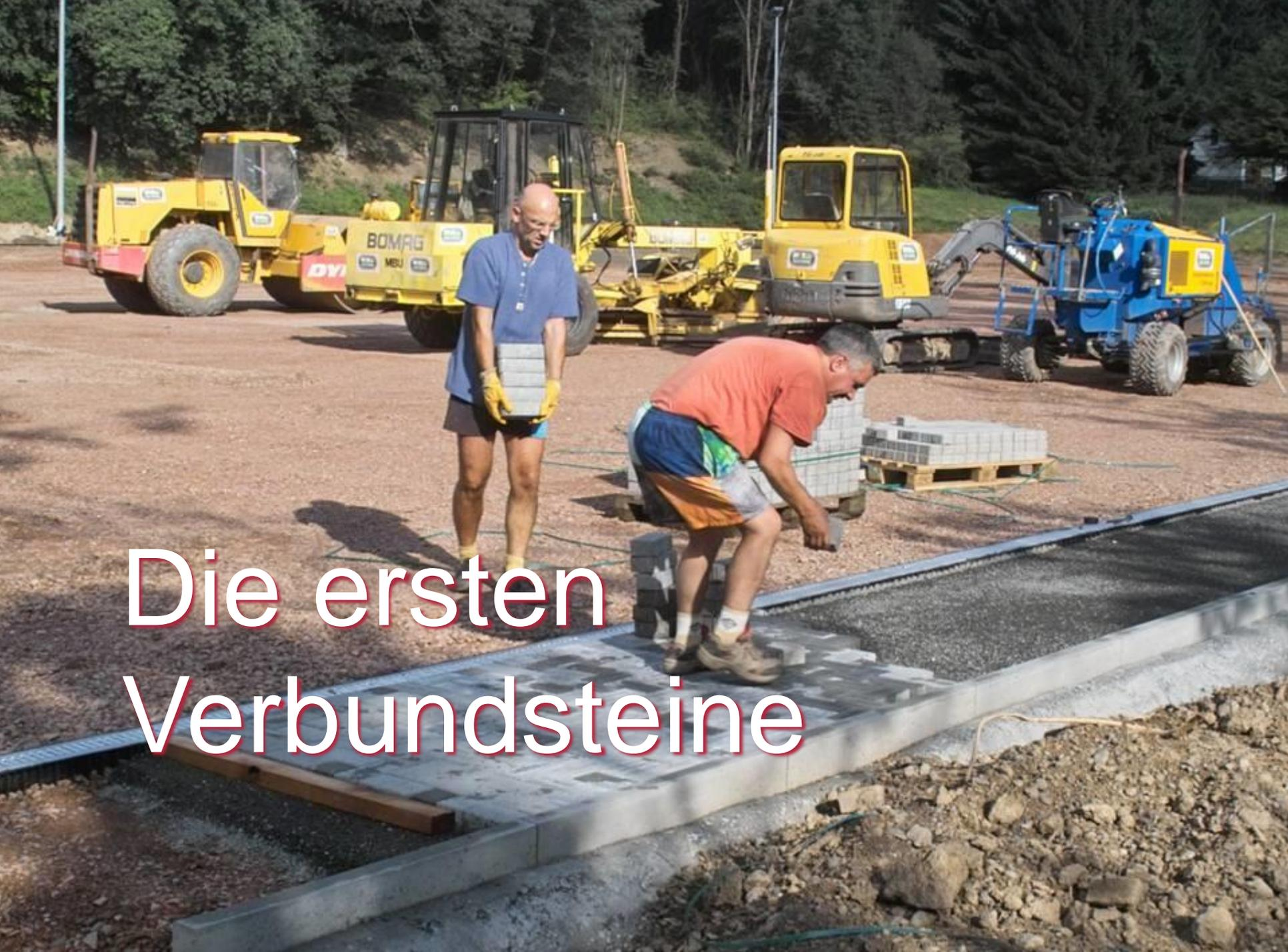
A construction site showing two workers laying interlocking concrete blocks in a trench. One worker in a blue shirt and yellow gloves carries a tray of blocks, while another in an orange shirt and blue shorts is kneeling to place them. In the background, there are yellow BOMAG and DYI machines, a blue tractor, and a pallet of blocks. The ground is covered in gravel and dirt.
